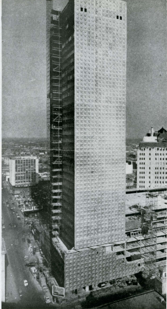
Republic National Bank Building
